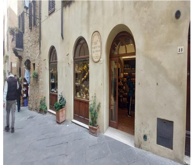
10 commercial premises along Corso Rossellino
