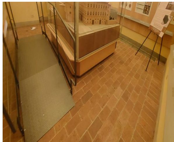
53 ramp metalliche internal
