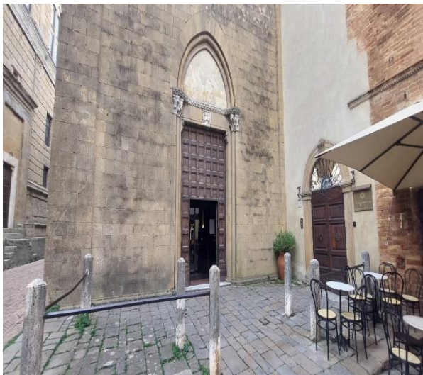
13 entrance portal of the church of S. Francesco with step
